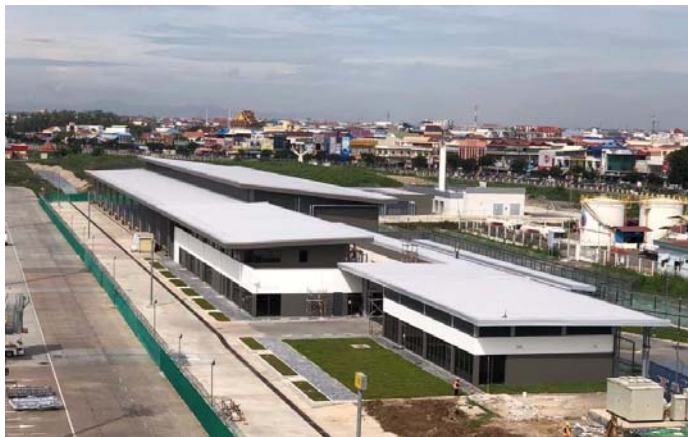
New Ground Handling Building Project at Phnom Penh International Airport, Civil and Structural Works Package for Cambodia Airport, Main Contractor : VINCI Construction Grands Projets
