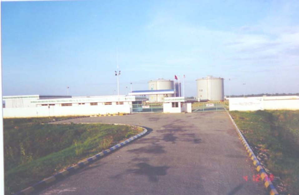
Petronas Terminal Project National Road No.1 (Choy Dang)
