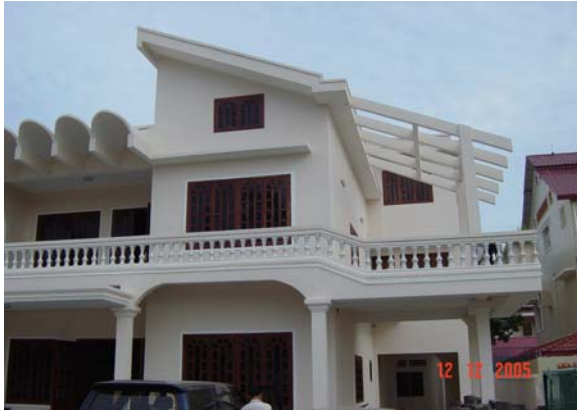
Villa Renovation Project, Road 315, Tuolkok, Phnom Penh Owner: Cambodia Brewery Limited
